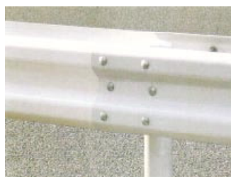
“Powdax Kino No. 3 SC” coating (left part of guard rail)
